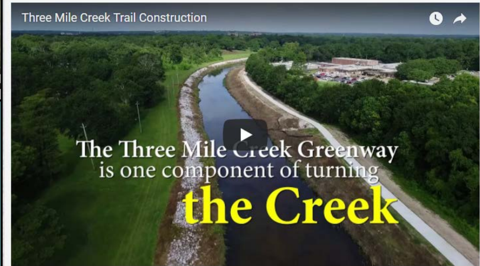
Three Mile Creek Trail Construction
