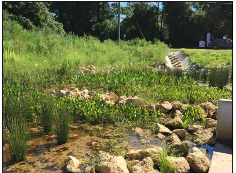
Spanish Fort stormwater retention pond across Highway 31 from Westminster Village.
