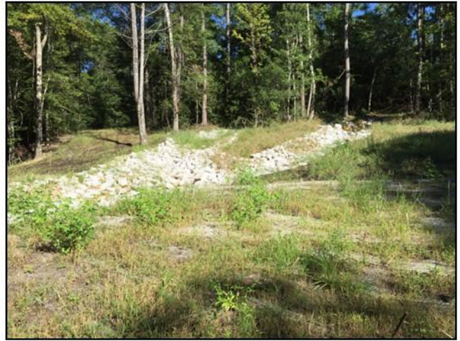
Rock used to stabilize a hillside steep impacting tributary segments J4-2 and J4-1.
