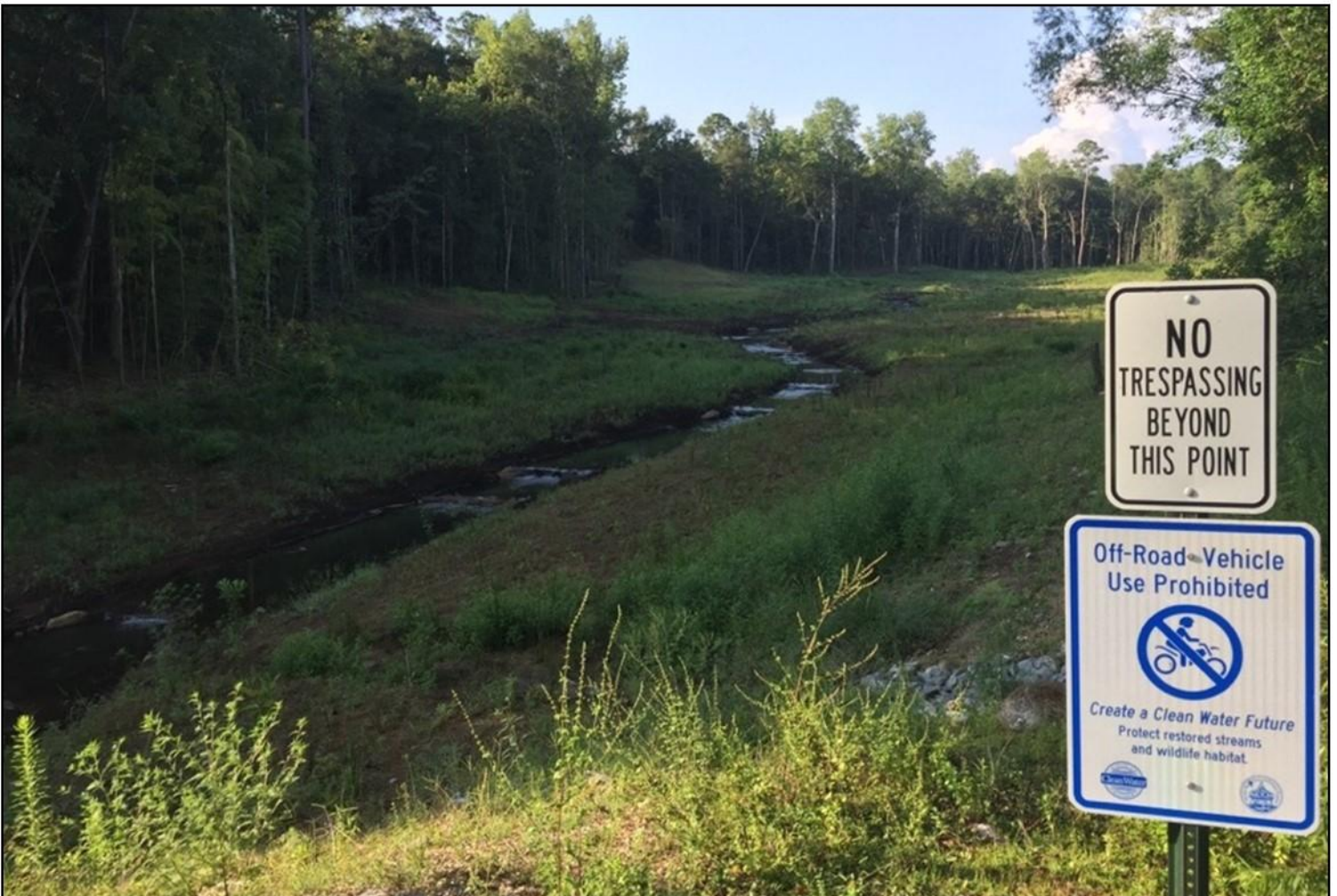
Tiawasee Creek tributaries TC1, TC2, & TC2-trib. This forested stream accommodated increased flows from residential and commercial development by eroding. Prior to restoration in early 2016, a total of 1,724 linear feet of tributaries delivered an average of 1,440 tons of sediment downstream each year due to headcutting, incision, and widening.
