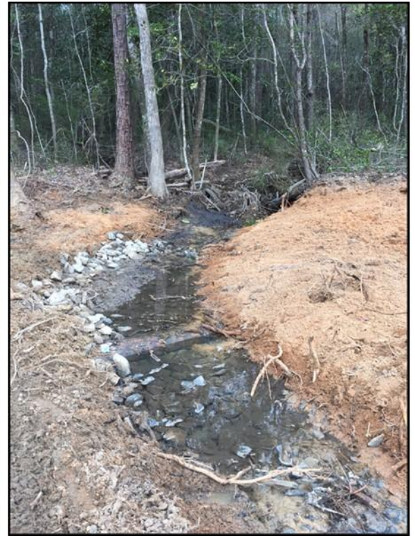
Tiawasee Creek tributaries TC1, TC2, & TC2-trib. This forested stream accommodated increased flows from residential and commercial development by eroding. Prior to restoration in early 2016, a total of 1,724 linear feet of tributaries delivered an average of 1,440 tons of sediment downstream each year due to headcutting, incision, and widening.
